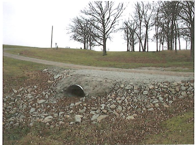
New Pipe Culvert
