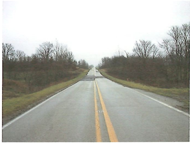
Patching of Existing Bituminous Surface
