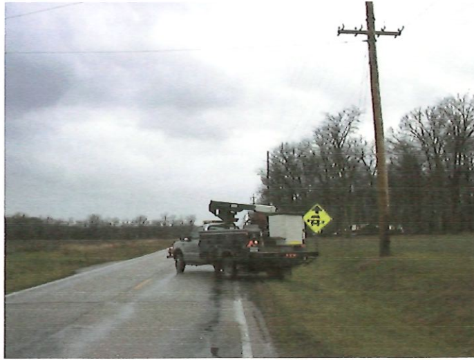
COMPLETED SIGN UPGRADE GRANT INSTALLATION
