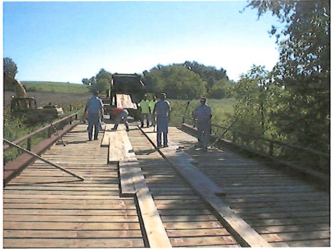
Deck Repair for Lakewood & Dry Point Townships
