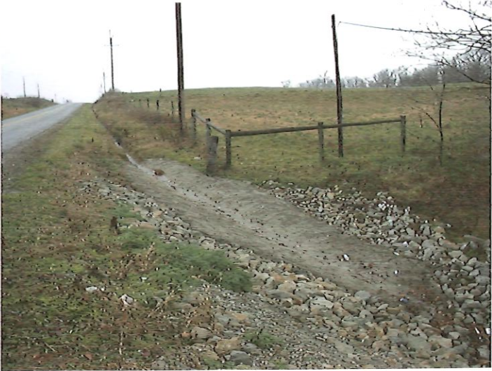
Repaired Gutter
