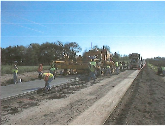
Placing Concrete Surface
