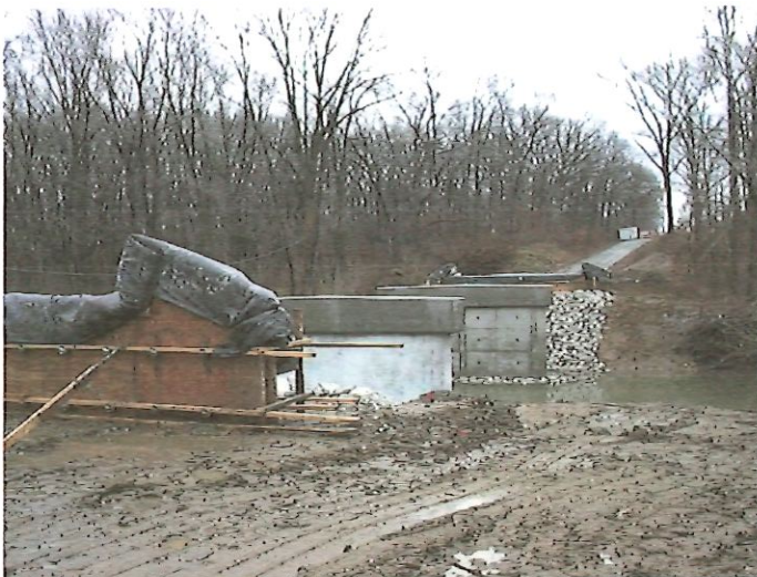
Bridge Construction in Progress
