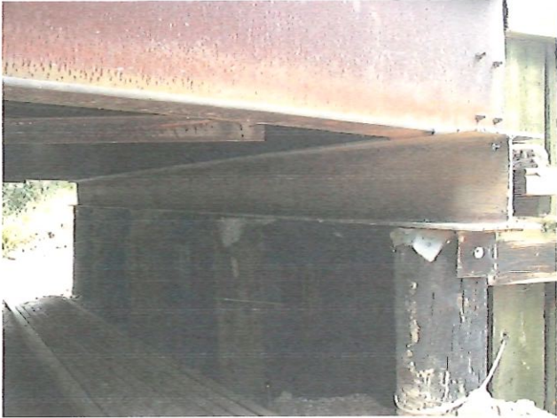
Bridge Repair in Cold Spring Township
