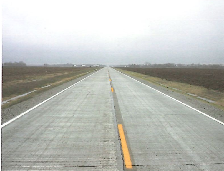
Finished Concrete Surface
