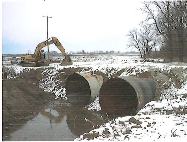
Tank Car Installation in Progress
