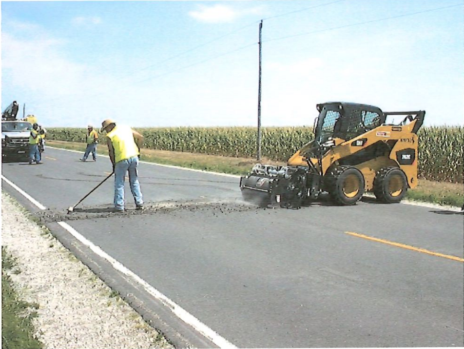
Surface Repair on Findlay-Assumption County Road
