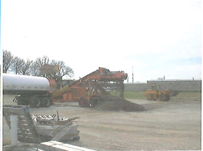
Make Cold Mix for County and Townships - 2500 tons
