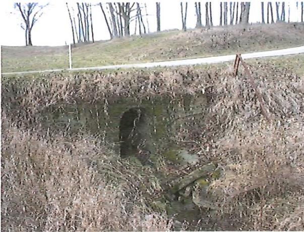
Existing Box Culvert
