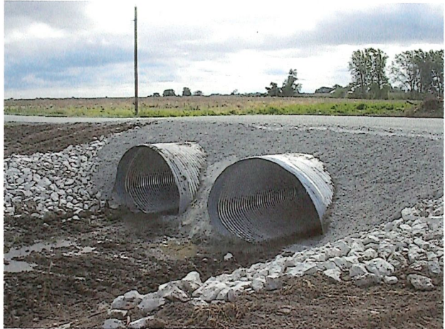
New Pipe Culverts
