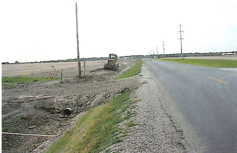
Ditch Cleaning along Oconee-Nokomis Road
