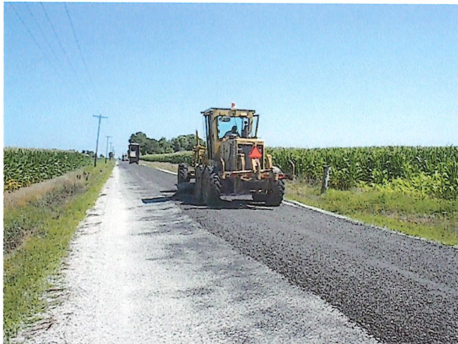
Cold Mix Overlay Findlay-Bethany Road
