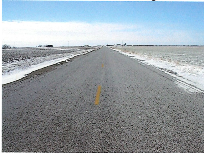
Finished Road Repair
