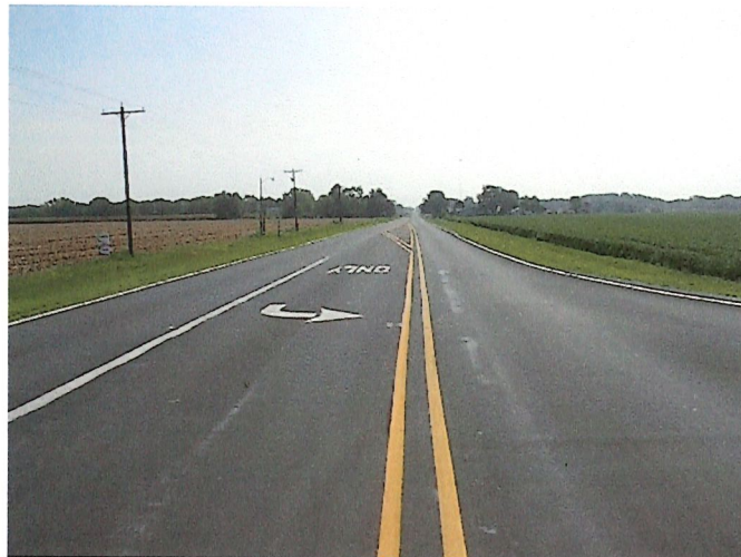
Finished Road Repair
