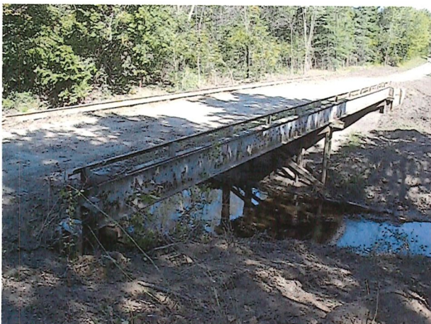
Old Bridge (5 ton)
