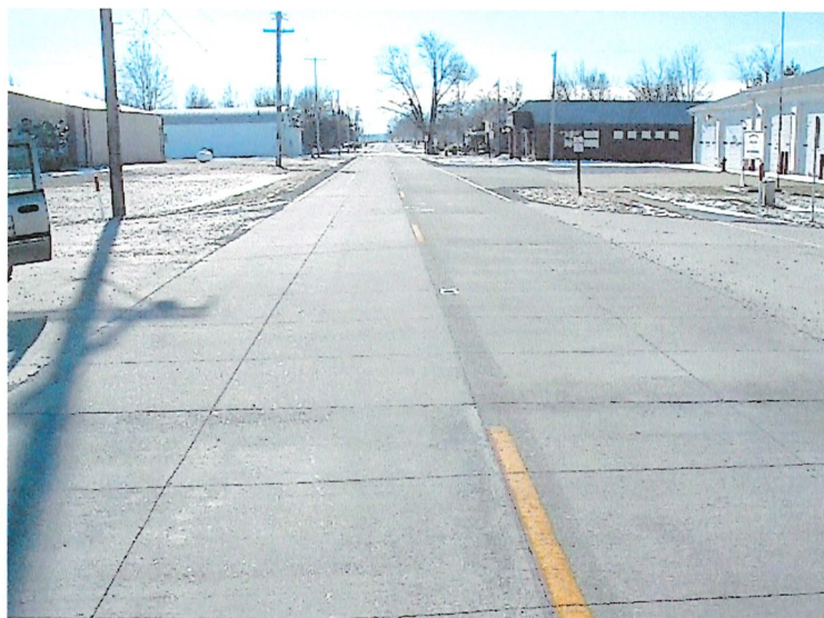
Finished Road Improvement
