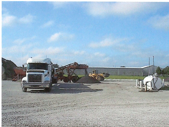
Make Cold Mix for County and Townships - 2900 tons (Most Ever)
