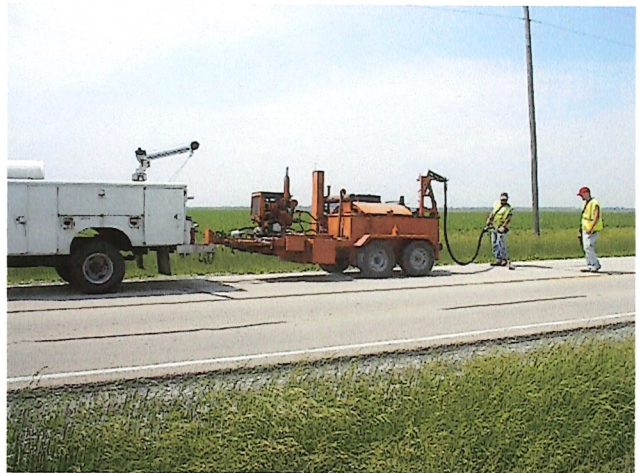
Crack Sealing Findlay-Assumption Road
