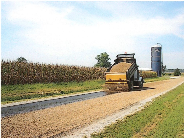
Seal Coat Clarksburg Road
