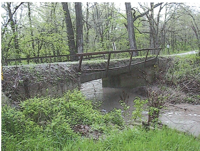
Existing Bridge (Closed)
