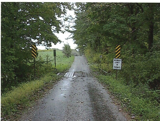
Existing Bridge (9 ton)
