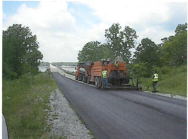
Microsurfacing of Road
