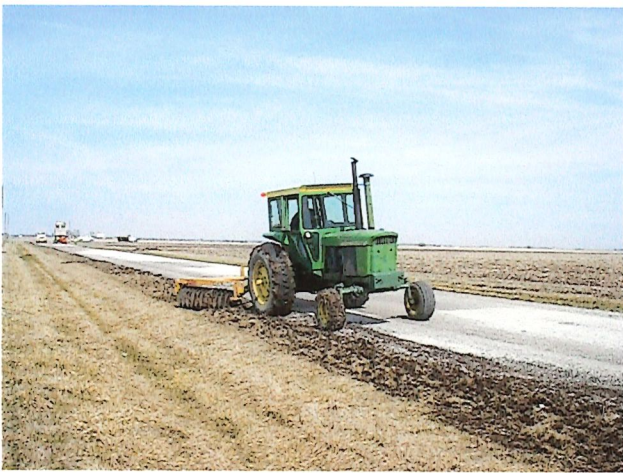
Shoulder Repair-Tower Hill-Moweaqua Rd
