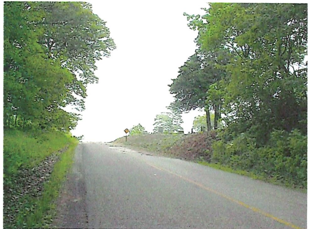
Brush Removal along Clarksburg Blacktop
