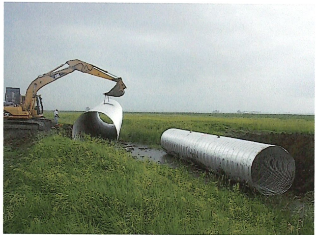
Installing 2 New Pipes
