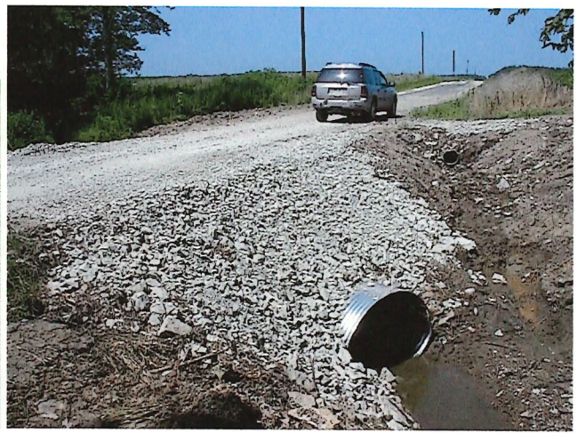
New Pipe Culvert
