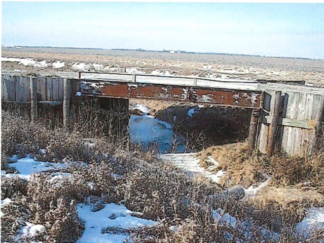
Existing Bridge (closed)
