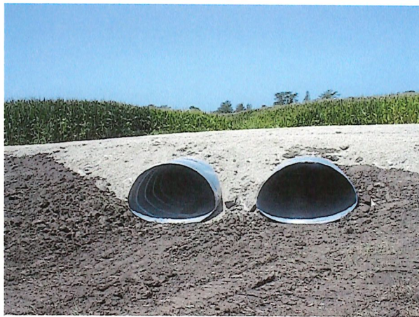
New Pipe Culverts
