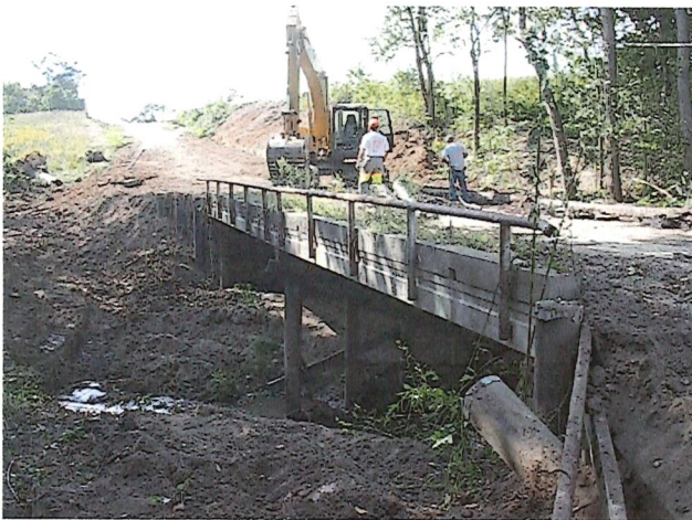
Old Bridge (Closed)
