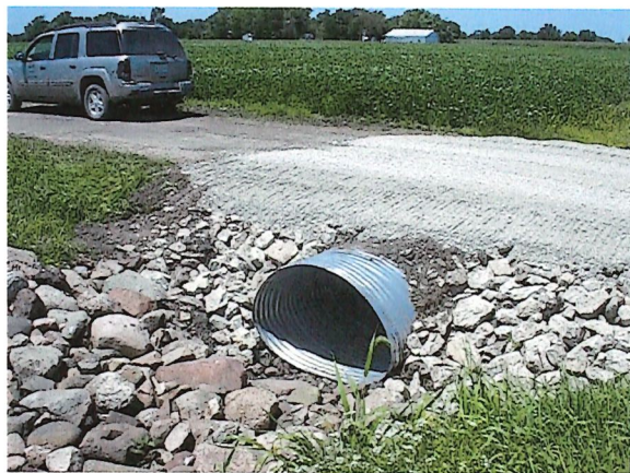
New Pipe Culvert
